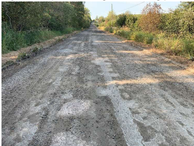
Figure 7: Required Clearing and Grubbing (Essex Rd.)
