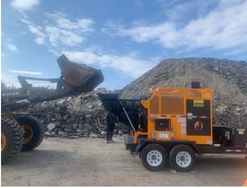
Asphalt recycler 1 ST bucket of old asphalt
