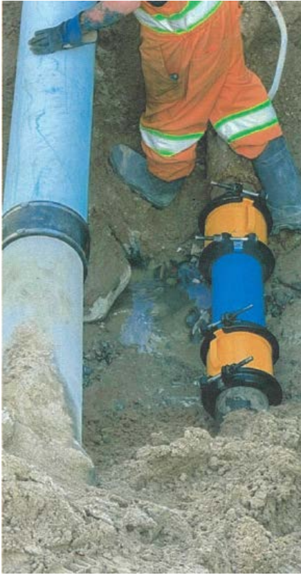
Gunne Crescent Repair
