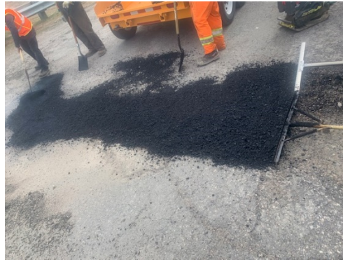
1 st patch of asphalt the roads crew laid.
