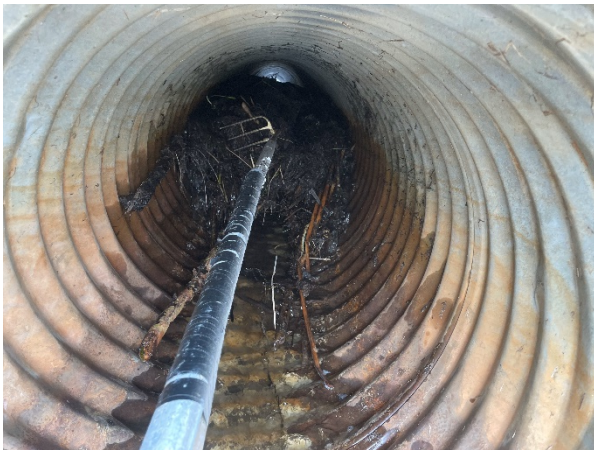
City and Contracted crews also got a handle on clearing beaver dam blockages near bridges and within culverts.
