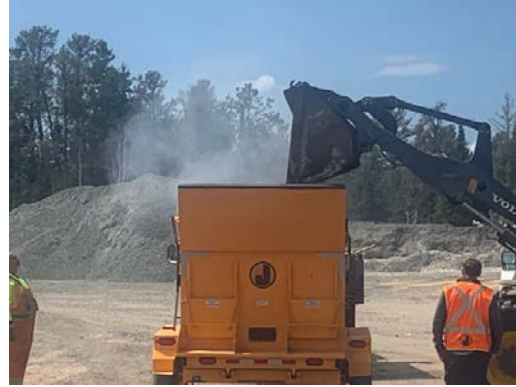
1 st bucket of hot recycled asphalt into the hot box
