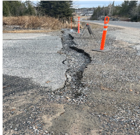
Steamed Culvert Barsky Crescent
