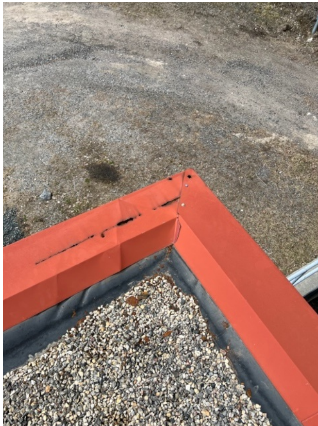
Roof and Flashing Repairs at the Wastewater Treatment Plant
