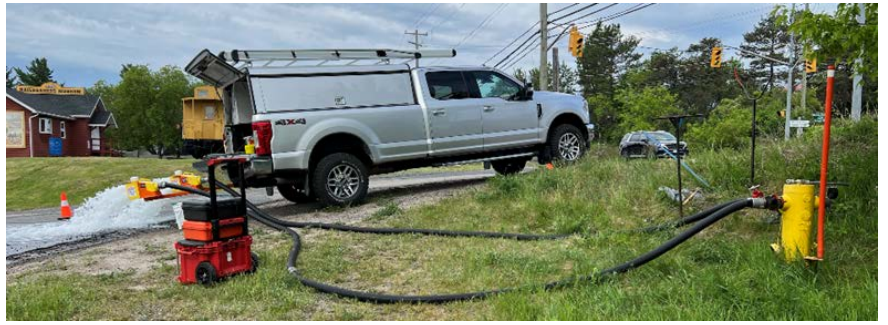
Wastewater Pump Removal
